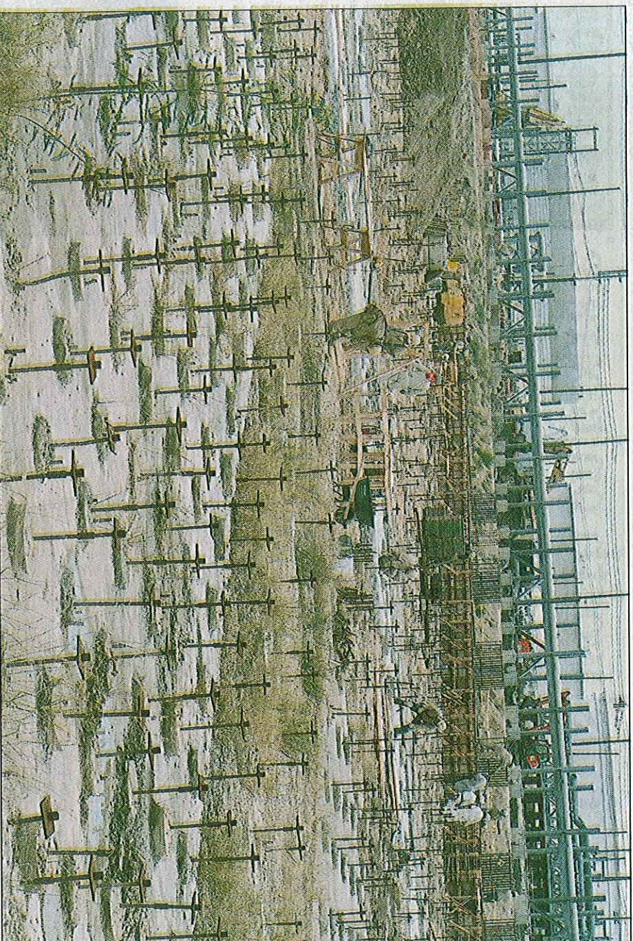
Concrete anchors jut from the ground as workers prepare the site for the hydrocracker unit.
